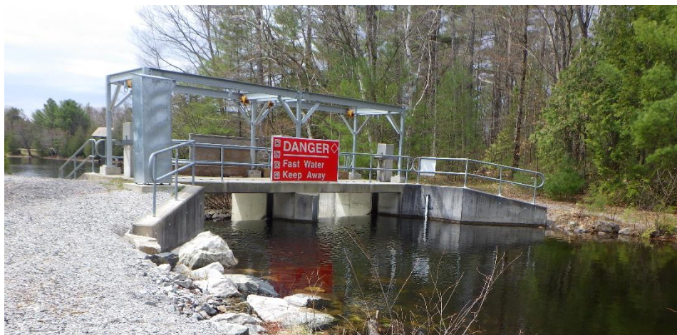
The dam and gauge at the outlet of Mazinaw Lake
